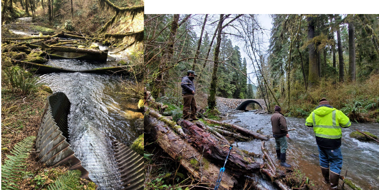
Figure 40. North Creek before (left) and after (right) culvert replacement.
