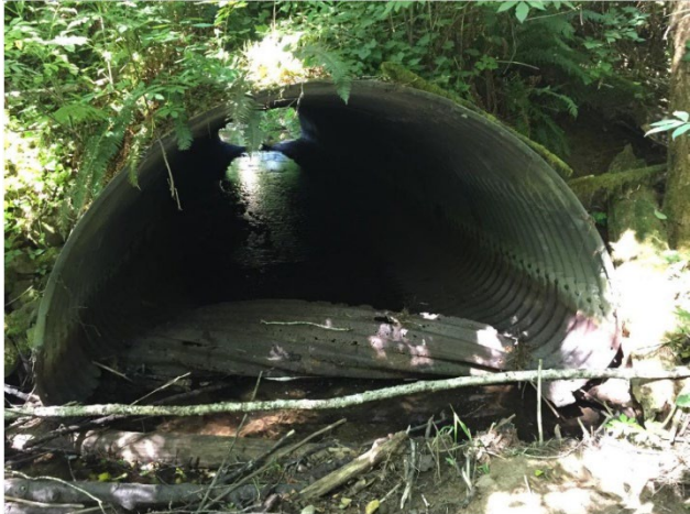
Figure 57: Cougar Creek Culvert
