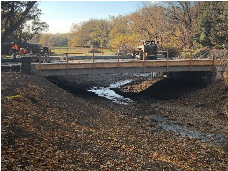
Figure 45: Wildhorse Creek after construction.
