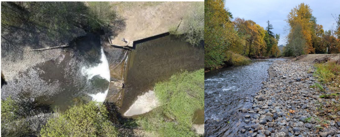
Figure 59: Balm Grove before and after.
