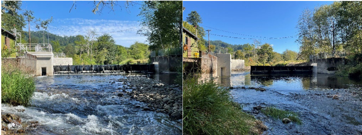
Figure 48: Cedar Creek before and after.
