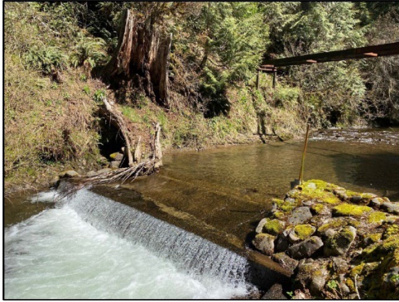
Figure 55: North Fork Eagle Creek Dam.
