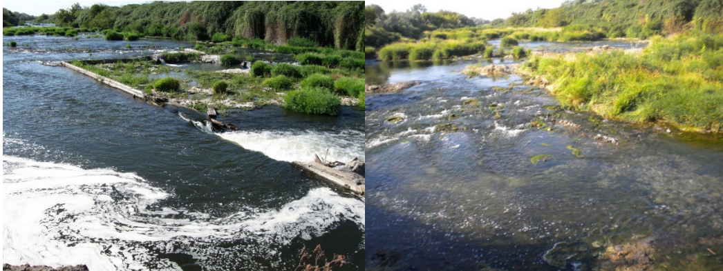
Figure 41. Brownell Dam before (left) and after (right)
